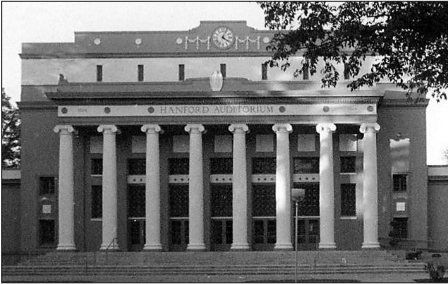
Hanford Civic Auditorium
